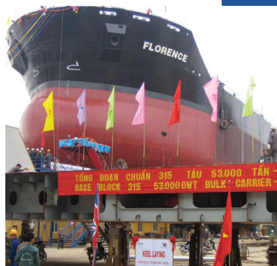
Launch of HL 01 'Florence' at Ha Long Shipyard and keel laying of HL02.
